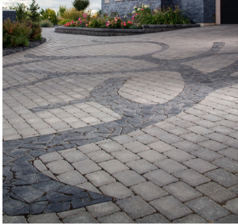
WALKWAY TO THE SEA PAVING
